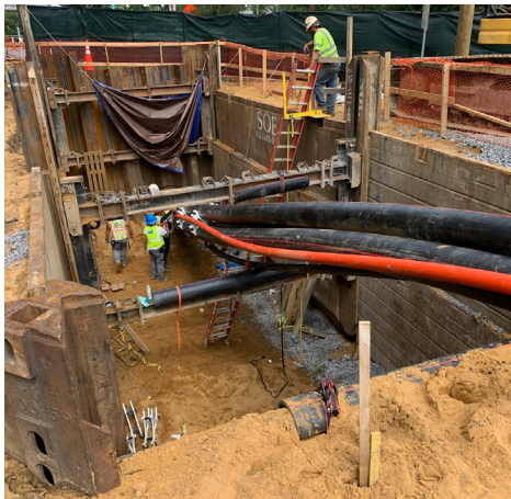
Top: Splice vault installation Middle: Utility crossing Bottom: Pullback during HDD
